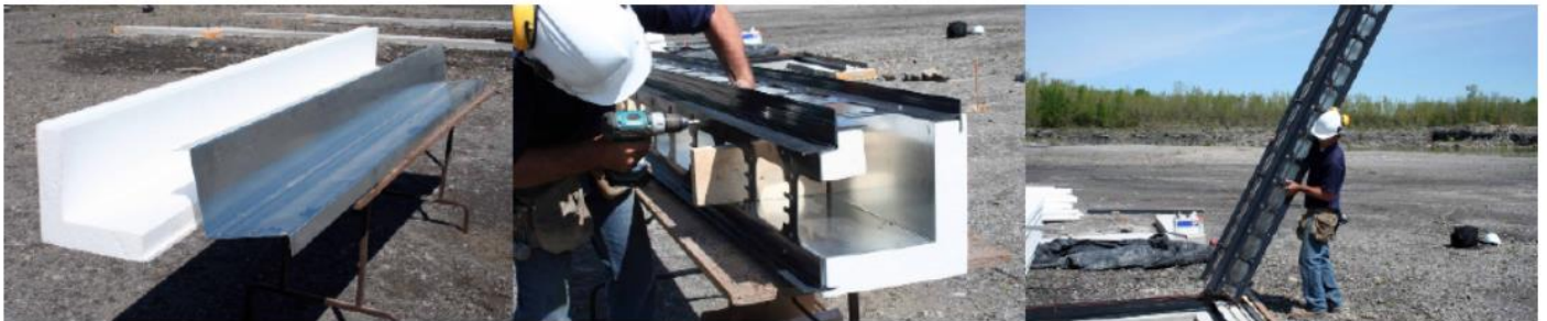
FIGURE 7 PERFORMED CORNER ASSEMBLY
