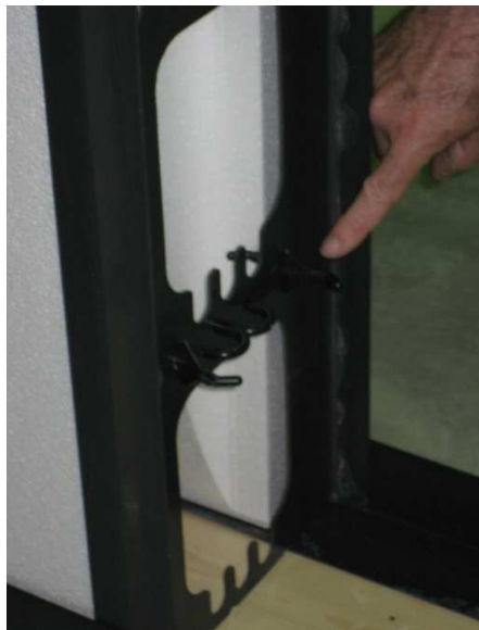
Figure 5. Furring Assembly and Retainer Clip
