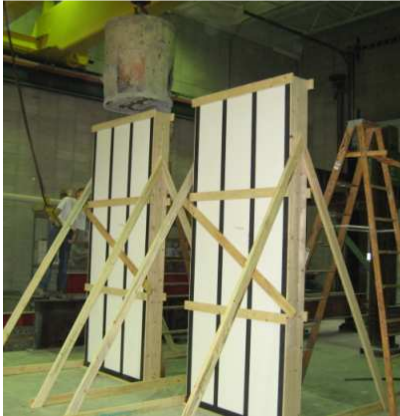
Figure 7. Constructed Wall Specimens
