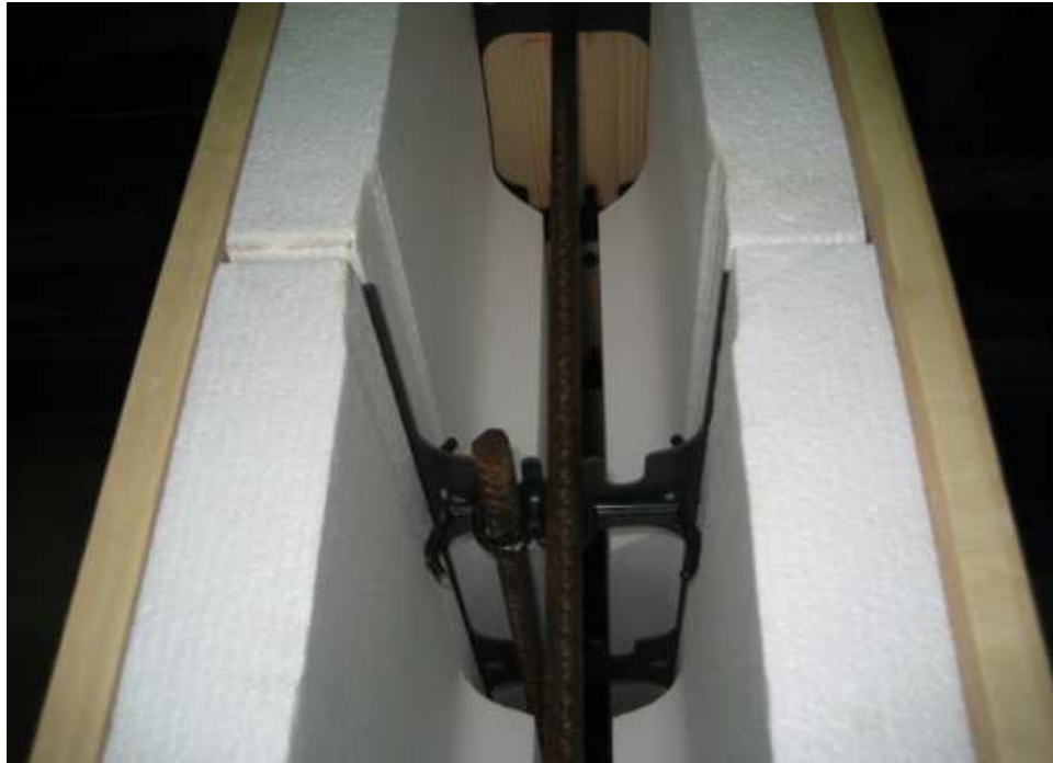
Figure 6. View of the Top Beam Formwork with Steel Reinforcement in Place
