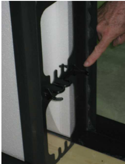
Figure 5. Furring Assembly and Retainer Clip
